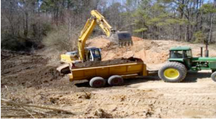
Contractor excavates waste from lagoon to spreader
